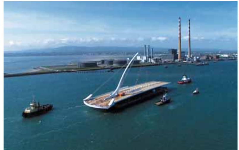
May 2009 – the Calatrava designed Samuel Beckett bridge is floated upstream into its position on the River Liffey.
